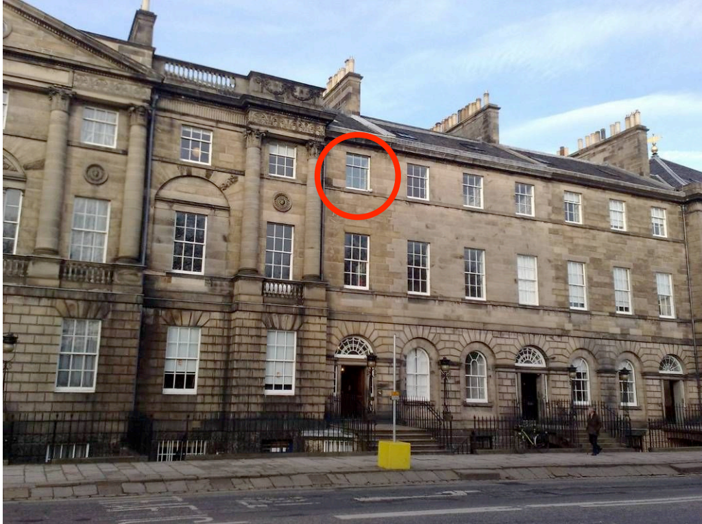
Figure 8 This window at Charlotte Square has new double-glazed sashes. The glazing bar dimensions are identical to the other windows. The new glass' reflective quality is slightly different, however this is minimal and is also dependent on light conditions and glass colour.
