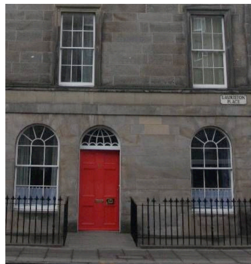
Figures 27 & 28 Appropriate double glazing (right; all windows are double-glazed) can be considerably more discreet than secondary glazing (left)
