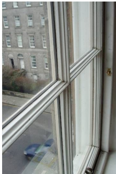
Figures 24 & 25 The thin spacer bar used in the left-hand image is very discreet. The thicker spacer bar in the right-hand image is more apparent when viewed at an angle
