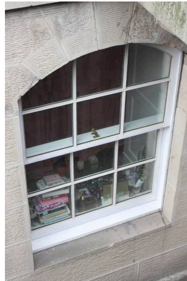
Figures 24 & 25 The thin spacer bar used in the left-hand image is very discreet. The thicker spacer bar in the right-hand image is more apparent when viewed at an angle
