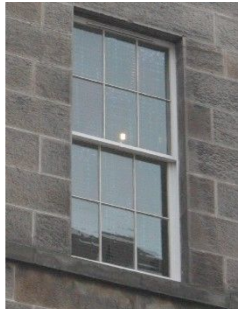
Figures 10 & 11 All these windows are now double-glazed. However, the bottom row of windows have Crown-effect outer panes (see right for detail)
