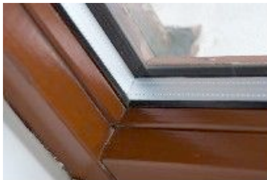
Figure 26 A typical metal spacer bar in a non-traditional timber frame
