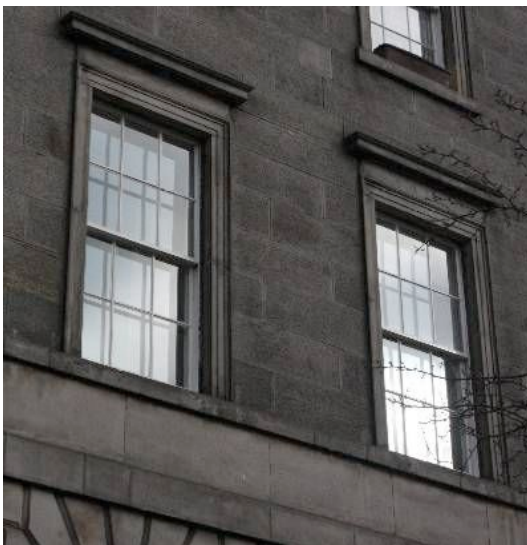
Figures 27 & 28 Appropriate double glazing (right; all windows are double-glazed) can be considerably more discreet than secondary glazing (left)
