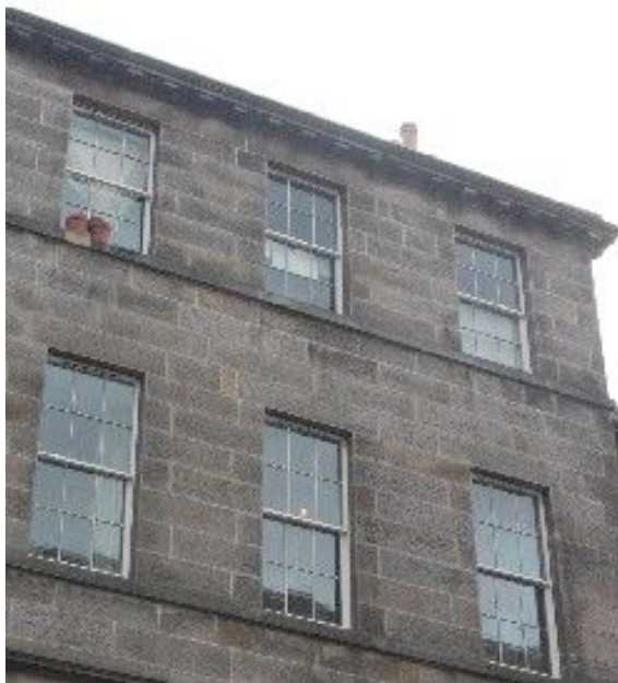
Figures 10 & 11 All these windows are now double-glazed. However, the bottom row of windows have Crown-effect outer panes (see right for detail)
