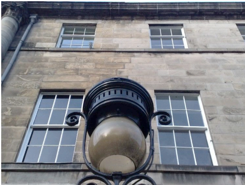
Figure 9 A closer view (top left), highlighting the discreetness that double glazing can achieve.
